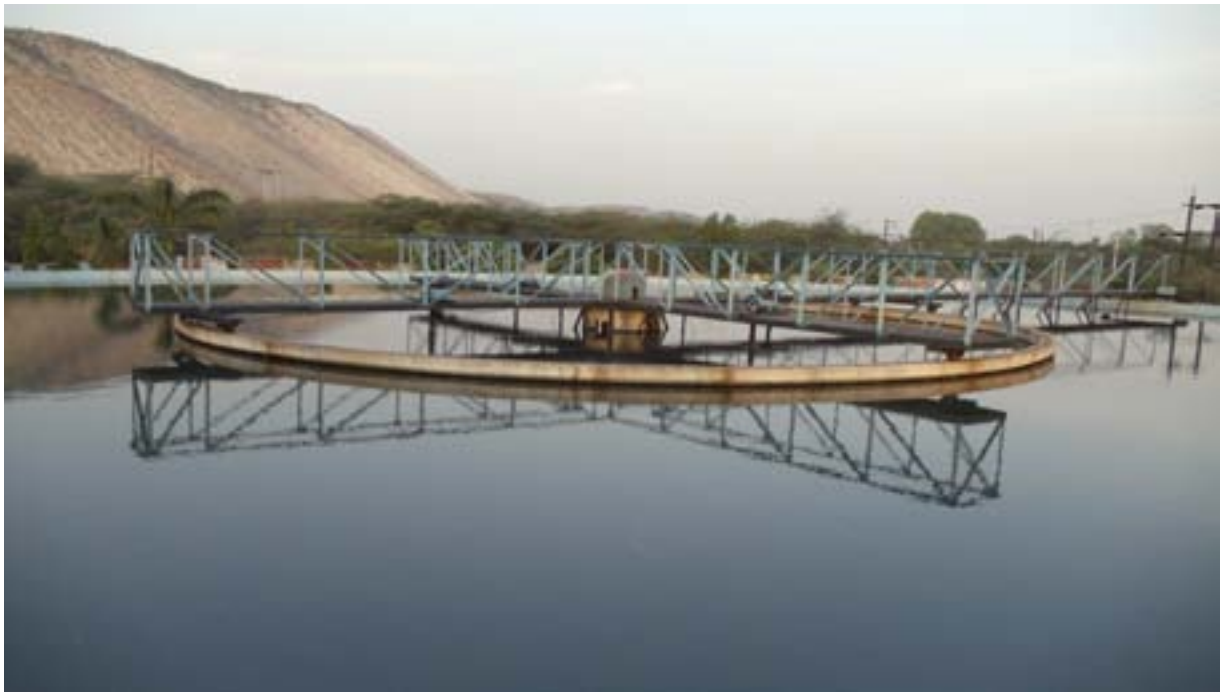
FIGURE 9 WATER TREATMENT PLANT AT KHADIA OPEN CAST MINE
